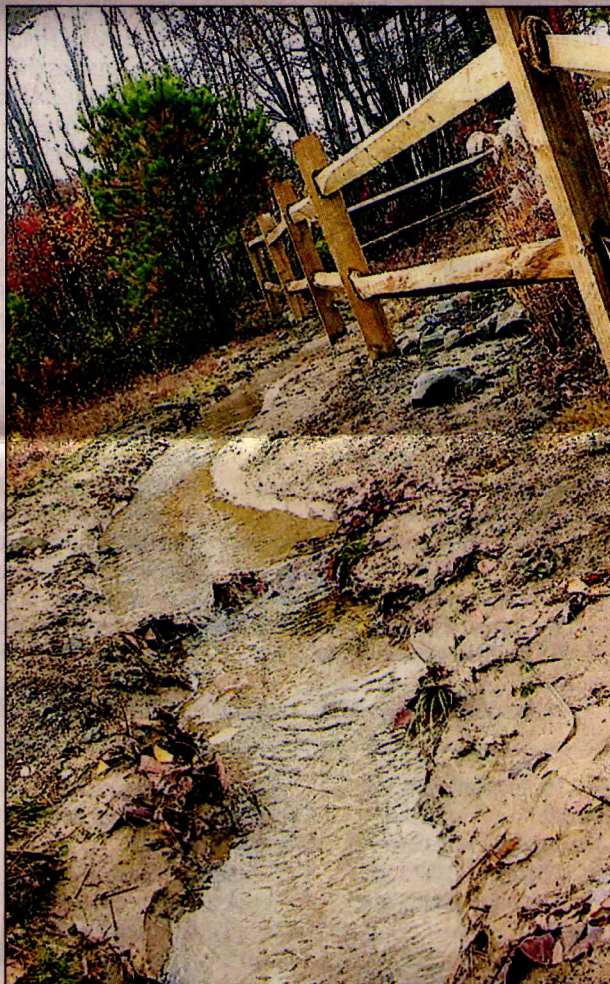
A trench moves water away from the Environmental Education Area at the Rails-to-Trails.
